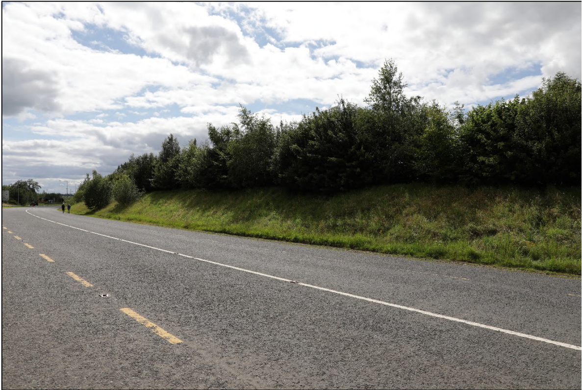
VIEW 10 – Existing from the R125 at Cooksland
