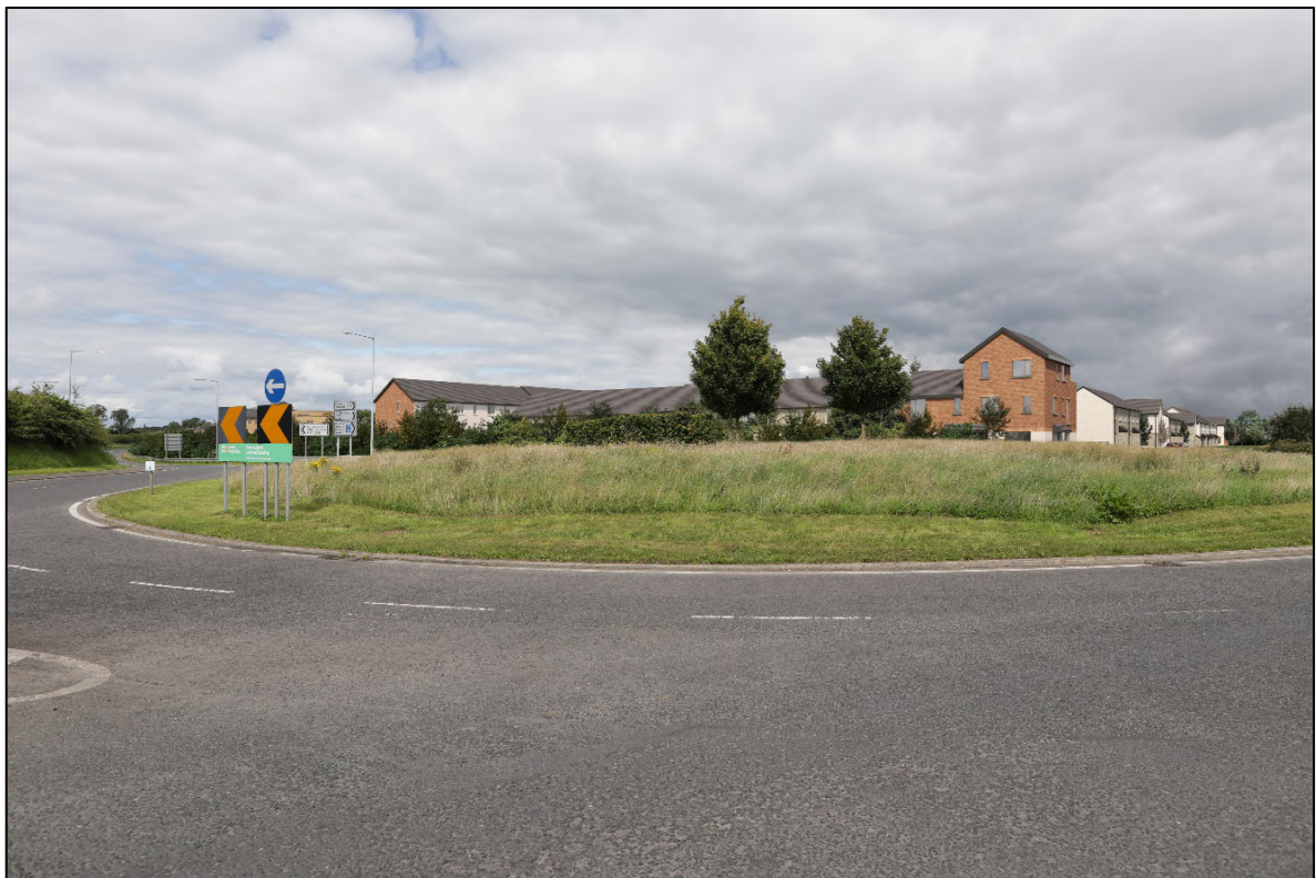
VIEW 03 – Proposed - Knockes Roundabout on R125
