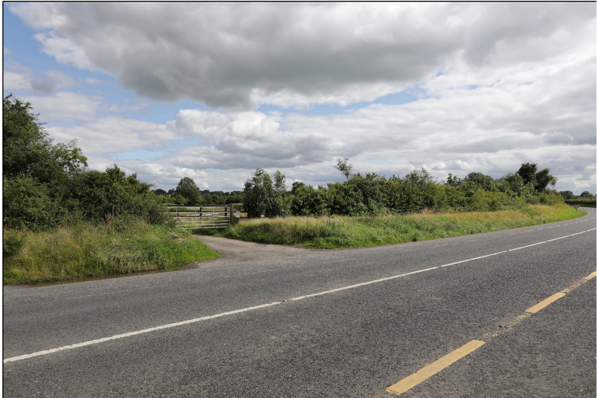
VIEW 07 – Existing from R125 Slip Road
